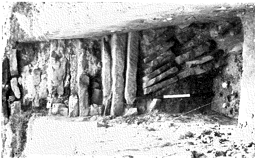
RETAINING WALL FOR EMBANKMENT Photo: G. Webster
