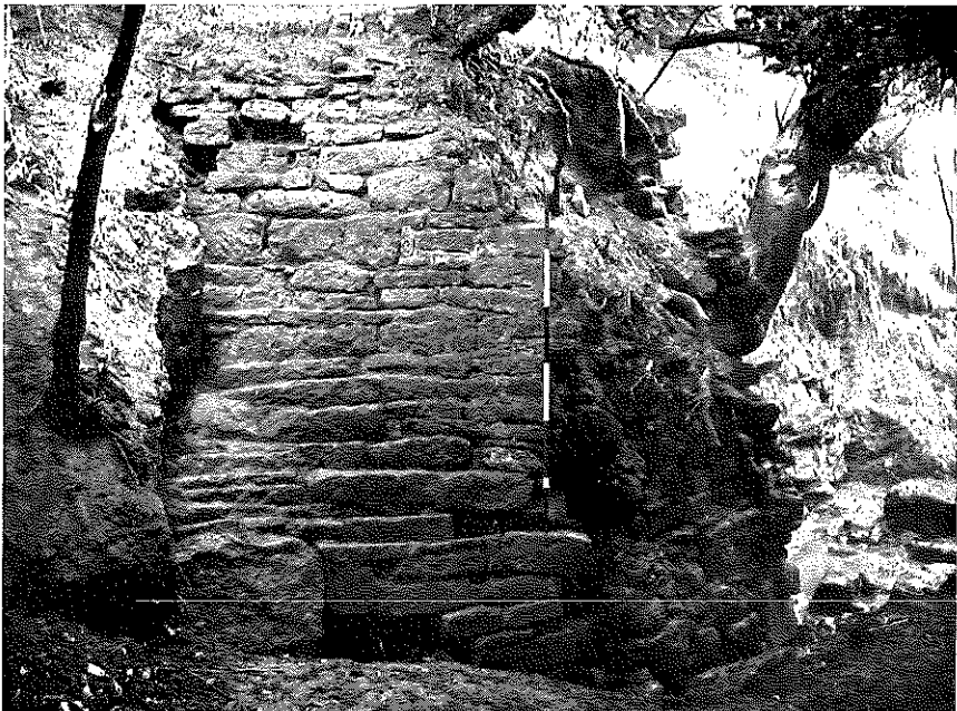
BRIDGE ABUTMENT, EAST FACE
