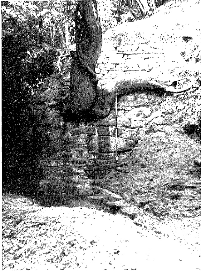
BRIDGE ABUTMENT, WEST FACE
